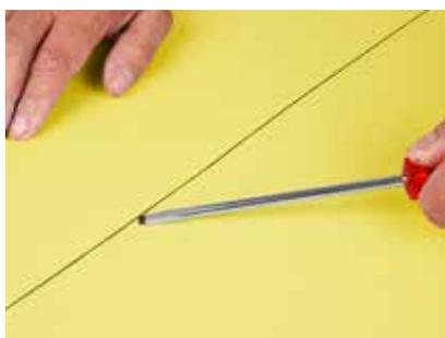
Visually checking with the aid of a broad screw driver to search for voids or misses at seam edges.
