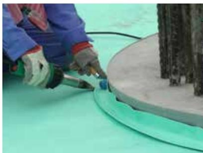
Handheld hot air welding gun and pressure roller, welding temperature adjustable. Suitable for single seam overlap weldings and detailing works, such as pile head connections or corners.
