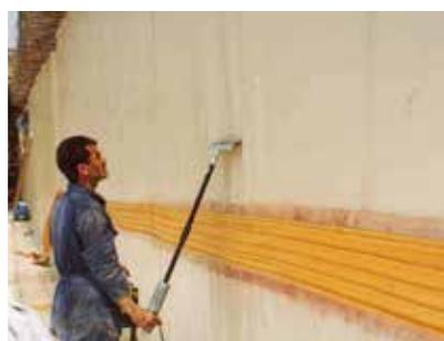
Area defect testing with an electrical copper wire brush. Electrical sparks signalizes capilarities in seams. Any defects in the membrane or at seam edges can be dedected, if an electrical conductor is placed underneath.
