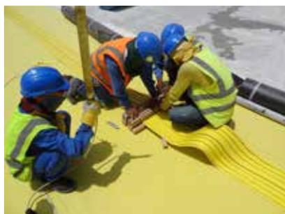
Butt-jointing of waterbars by welding with heating blade for creating compartments.
