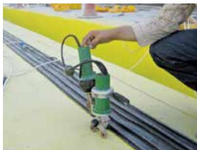
Semi-automatic hot air welding machine and pressure roller, welding temperature and welding speed adjustable. Suitable for single seam overlap weldings, detailing works and welding of waterstops on installed membranes.
