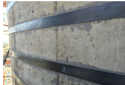
Contractor : Teichmann Structures
