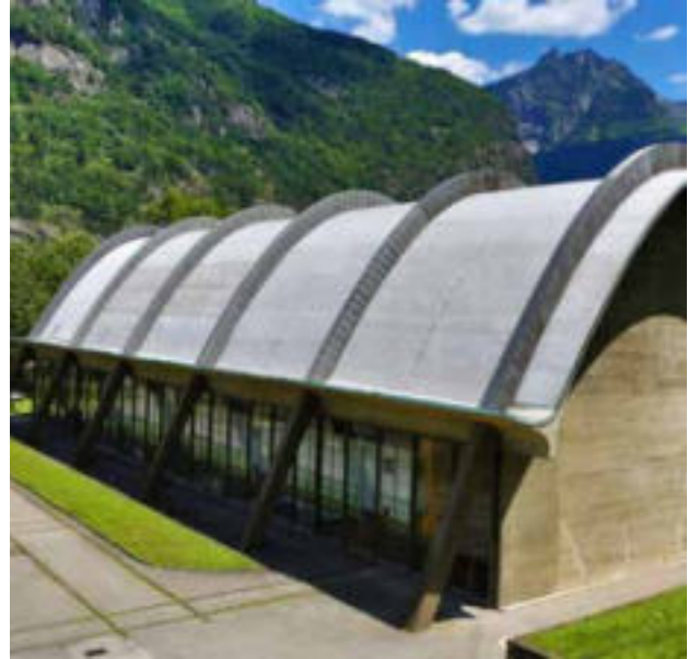
Project year: 1967 | Nuova Biaschina Hydroelectric Plant, Personico, Switzerland | Sarnafil® G 410-12
